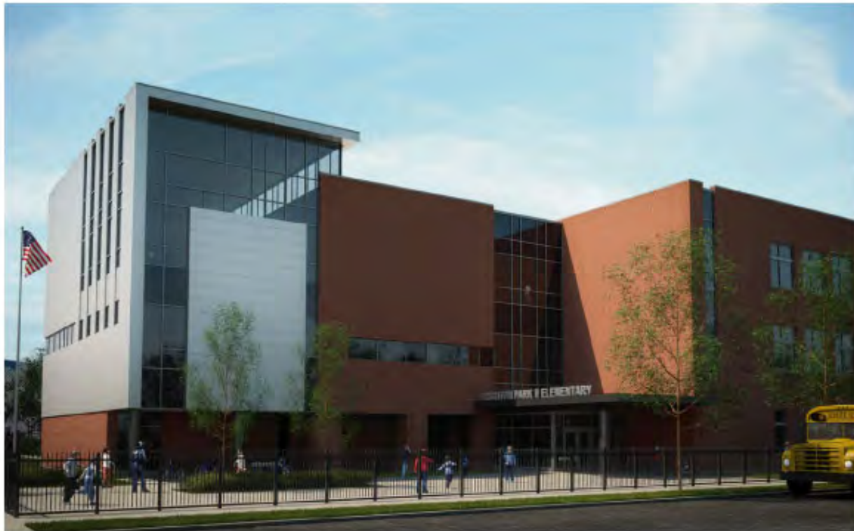
BRIGHTON PARK II ELEMENTARY SCHOOL
