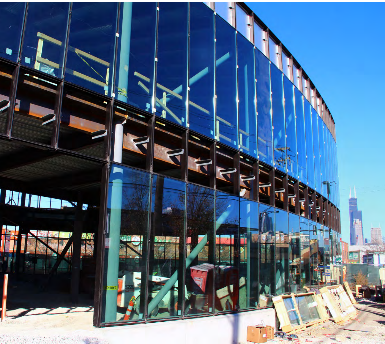
Construction at the Chinatown Branch Library.
