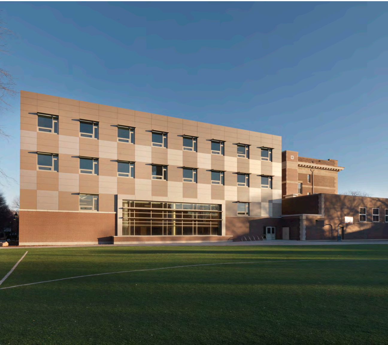
The new addition at Coonley Elementary School opened in September.
