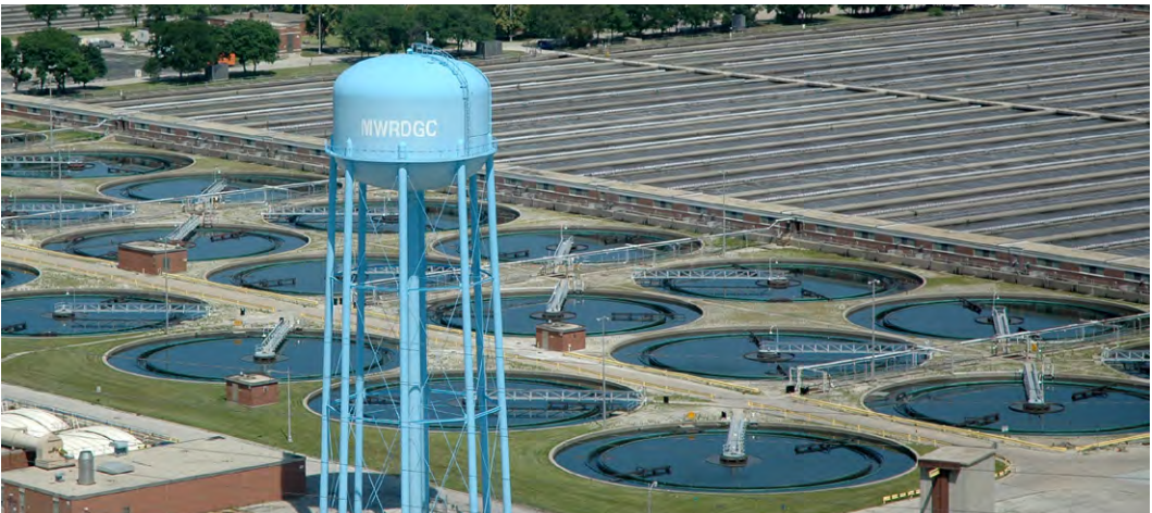
The MWRD's Stickney Wastewater Treatment Center.
