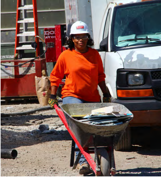
A worker pushes a wheelbarrow at the site of the Dunne Technology Academy modernization project.
