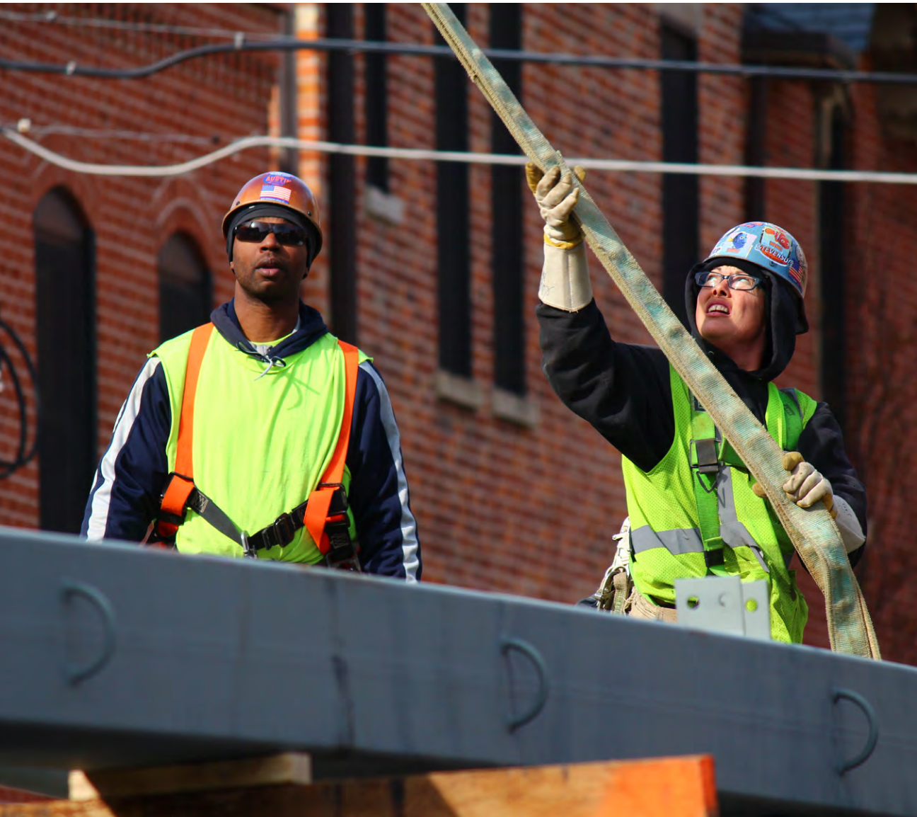
Workers at the Abraham Lincoln Elementary School Annex.
